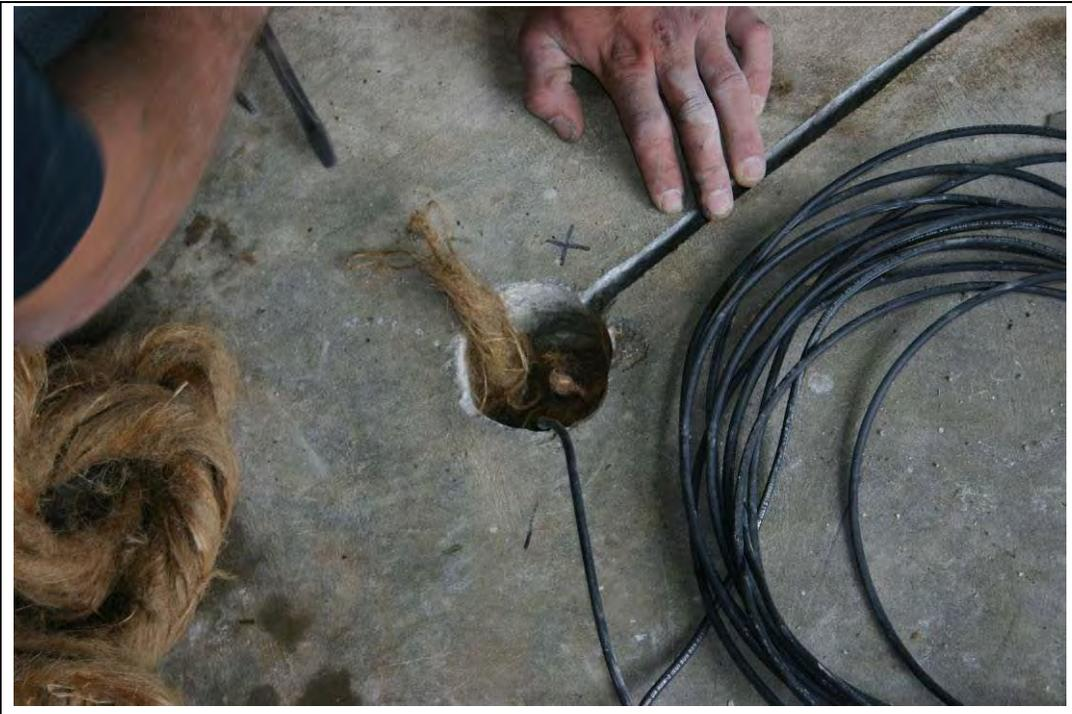
Figure E-12. Installation of oakum around a cathode.
