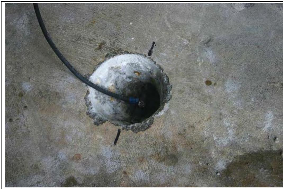
Figure E-16. Rebar lead wire connection.
