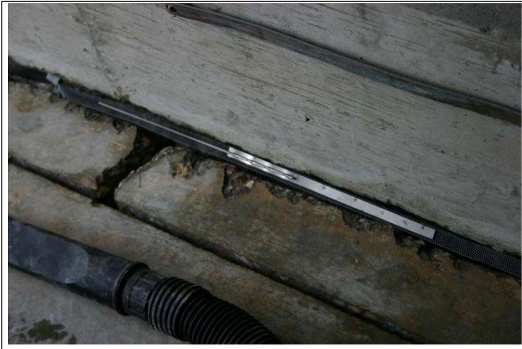
Figure E-9. Titanium wire connector welded to anode.
