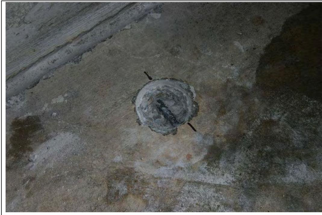
Figure E-5. Exposed rebar.
