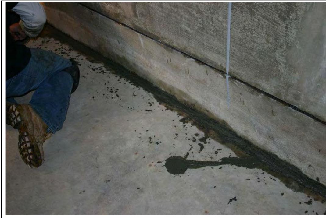
Figure E-15. Grout finish over cathode.
