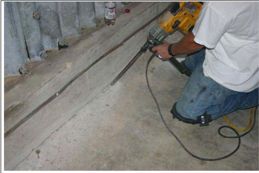
Figure E-3. Chipping of anode slot.
