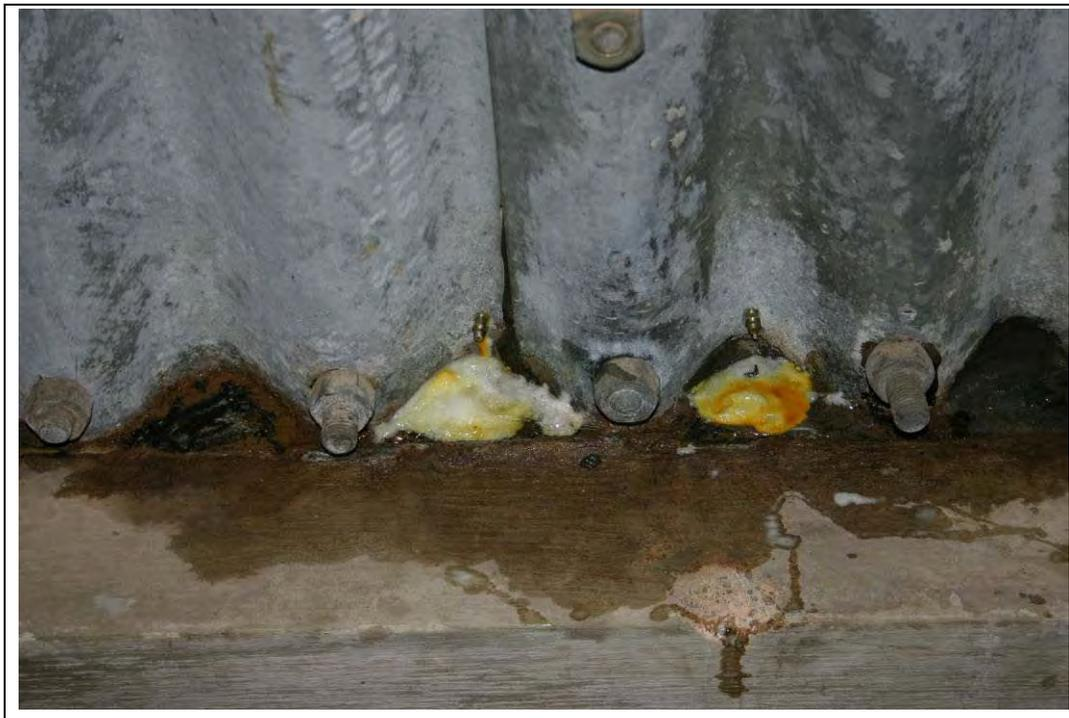
Figure E-27. Leak injection.
