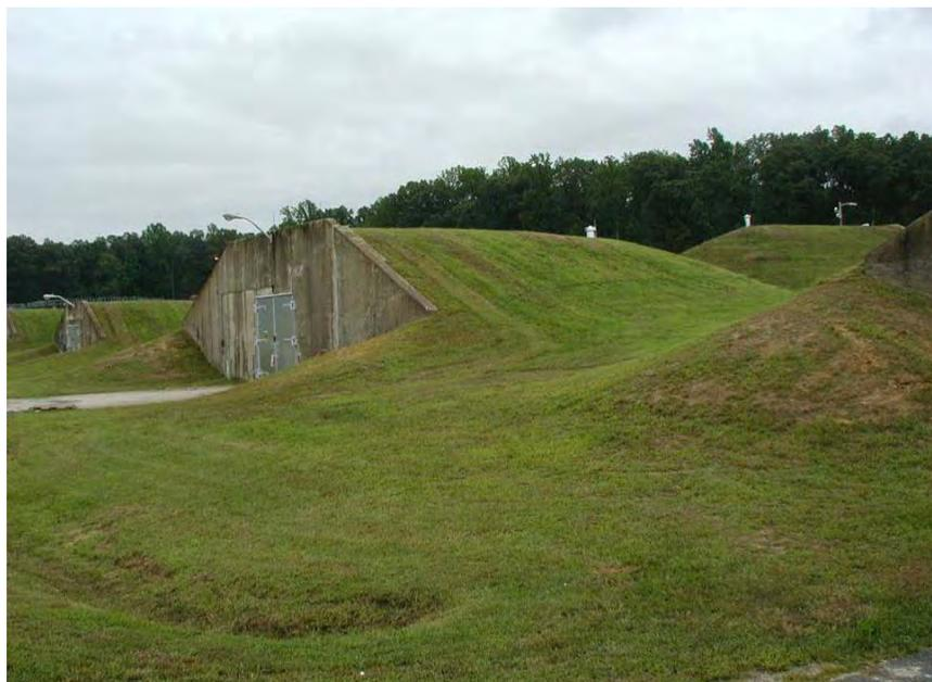
Figure 2.2. Typical steel arch earth-covered magazine.
