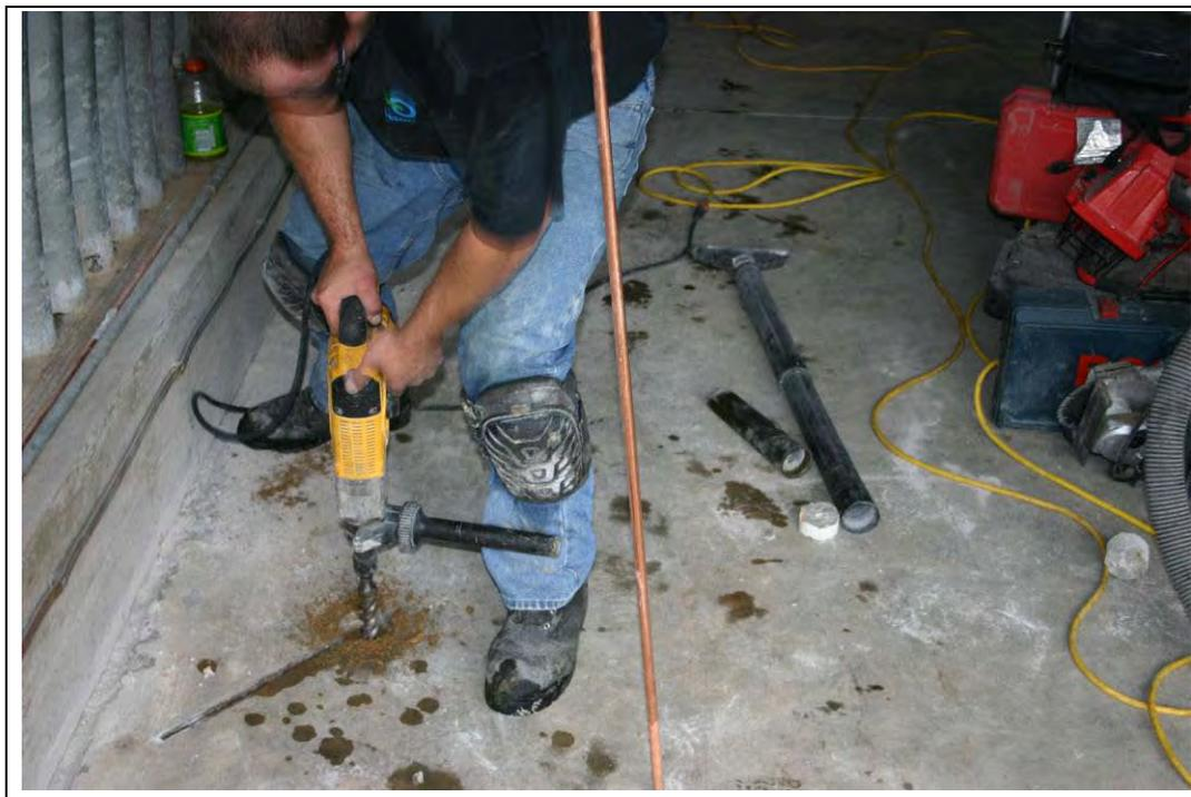
Figure E-4. Drilling of hole for cathode and cathode to be installed.
