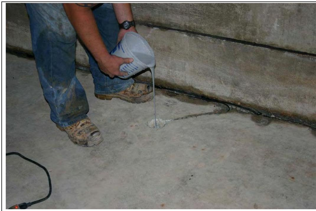
Figure E-14. Epoxy potting of cathode.
