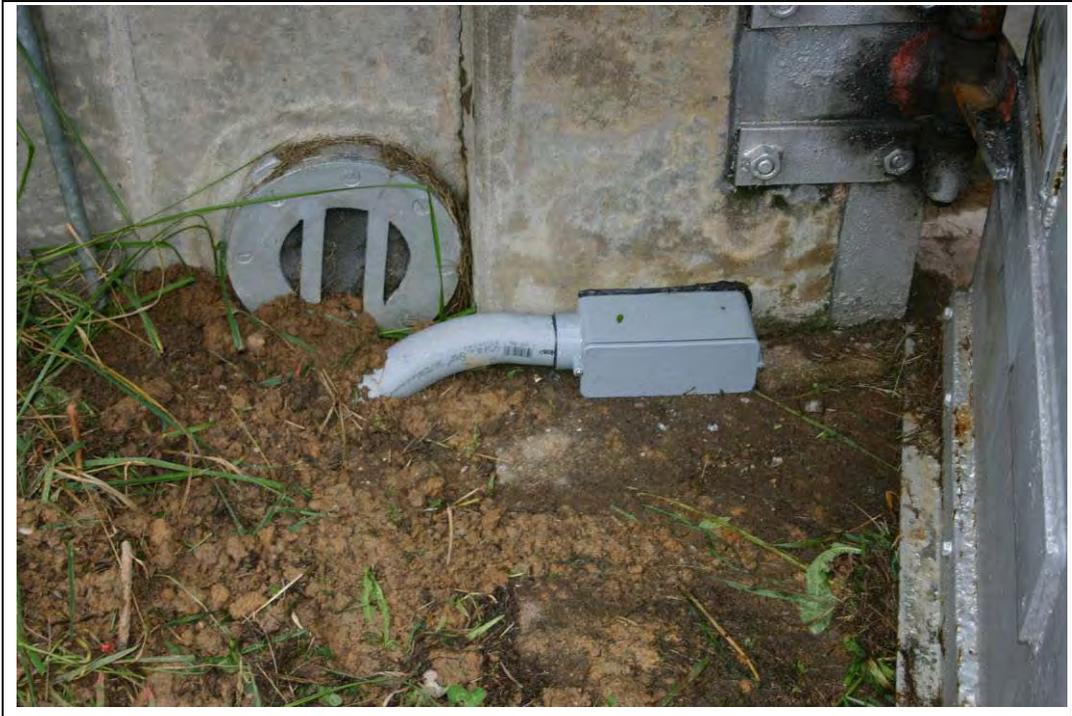
Figure E-20. PVC Conduit from magazine to connector box.
