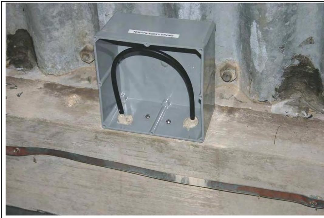
Figure E-45. Interior of EOP system relative humidity/temperature sensor wiring box.
