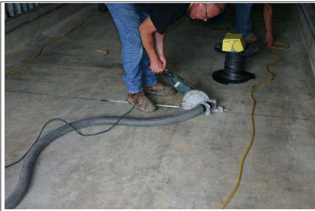
Figure E-2. Saw cutting of anode slot.
