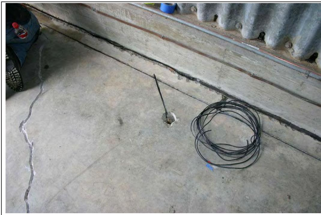
Figure E-6. Slot for lead wires.
