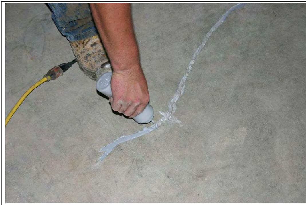
Figure E-8. Crack being filled with epoxy.
