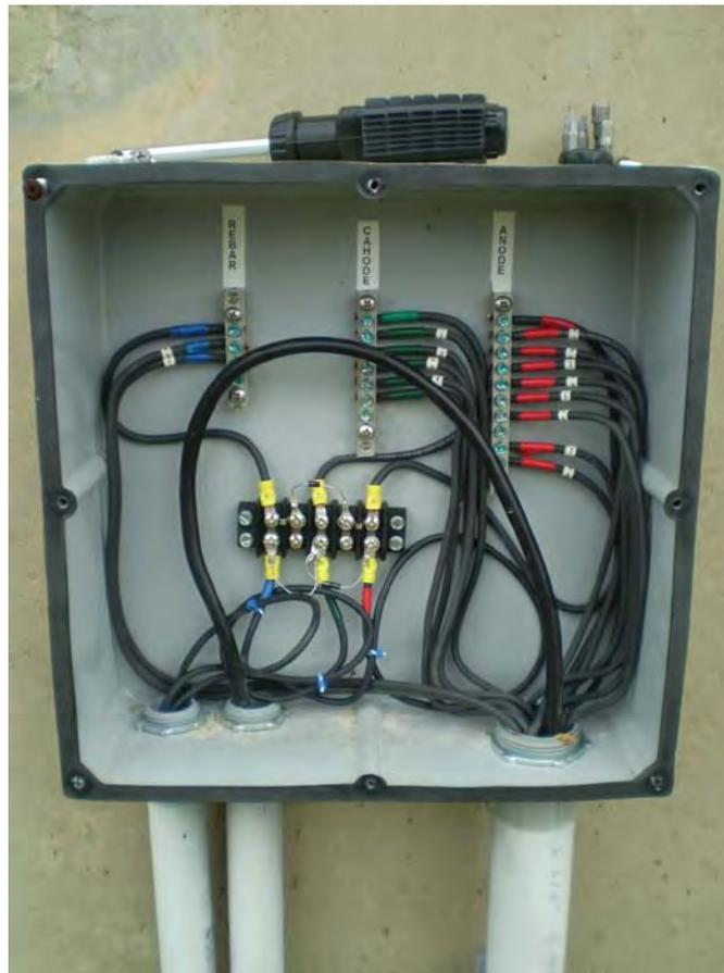
Figure E-58. Magazine connector box with MOVs installed.
